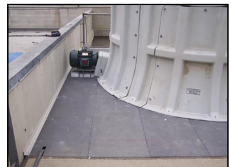
Concrete Structure with Fiberglass Deck
